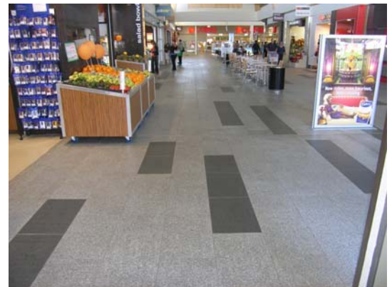
* First internal commercial application of exfoliated non-slip granite pavers.
